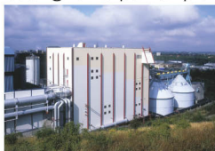
Högdalens combined heating- and power plant
