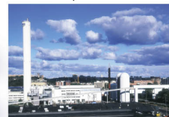
Hammarby thermal powerstation
